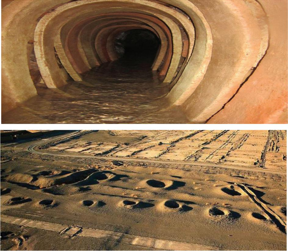
Fig.3.1.2 *Qanat* in the central plateau, and a row of openings of ventilation shafts
